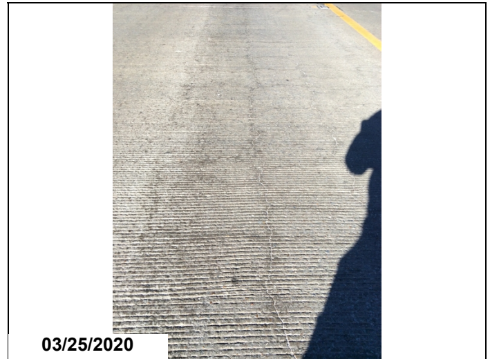
Longitudinal and transverse deck cracking.
