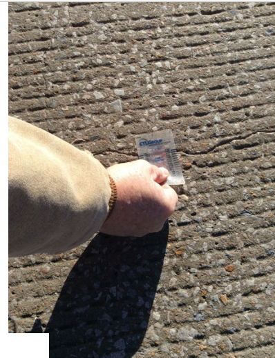
Deck cracking
