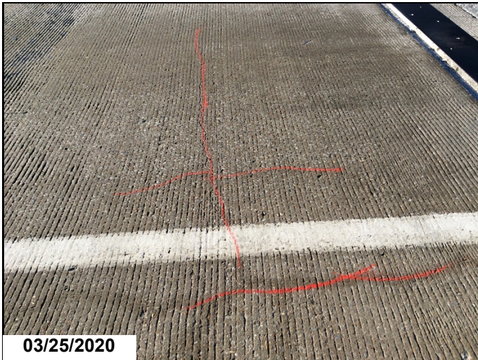
Span #1, Left lane-Transverse and longitudinal cracking.
