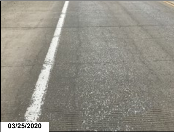
Deck surface Typical full-length longitudinal cracking
