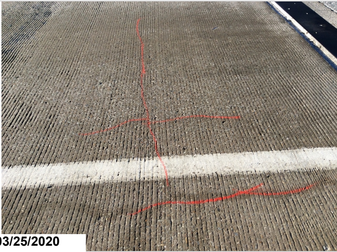
Span #1, Left lane-Transverse and longitudinal cracking.
