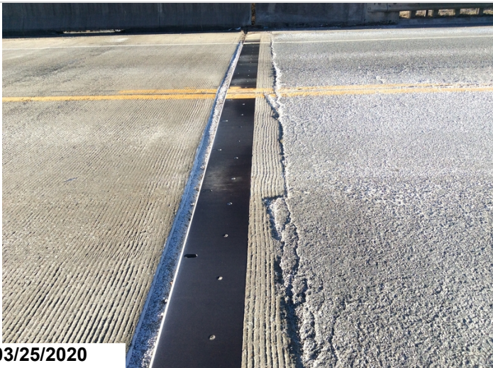
Abutment #1 has damage to the top of backwalls that appear to be from mechanical grinding.
