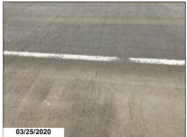
Deck surface typical transverse cracking.
