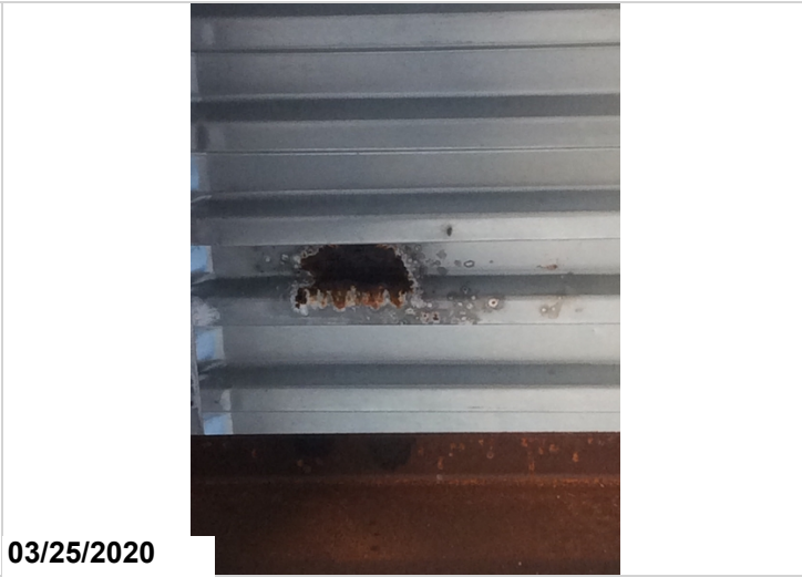
Span 5 has corrosion in span 5 bays 2 and 4.
