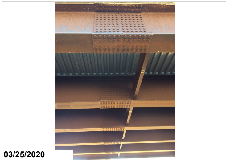
General view of splice plates in span 5
