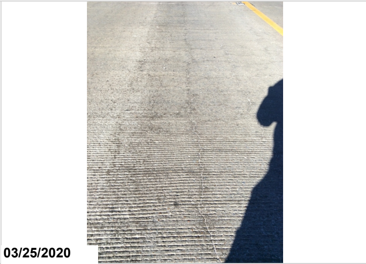
General deck cracking
