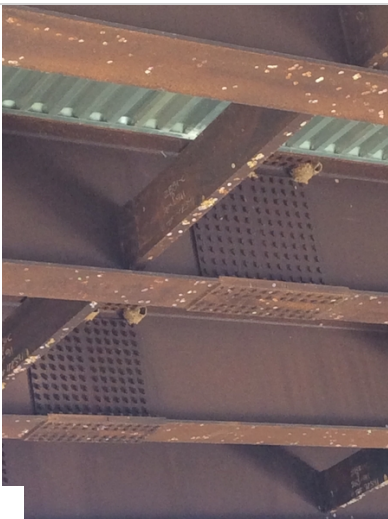
General view of splice plates in span 2.
