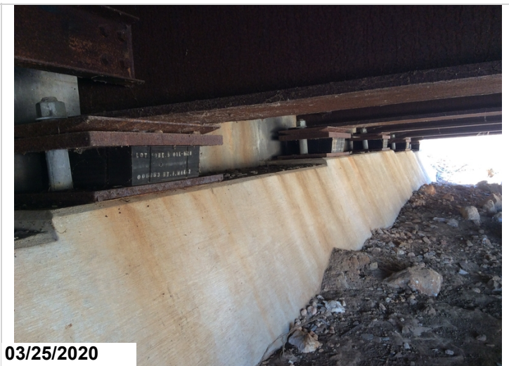
Abutment #2-General view of bearing devices.
