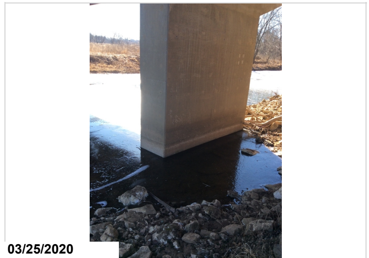
Bent one footing has cover
