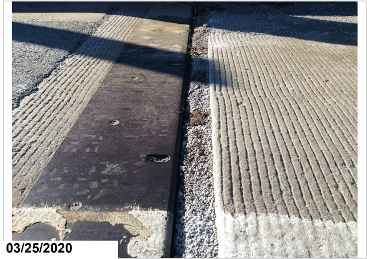
Abutment #2-Debris impact in expansion joint.
